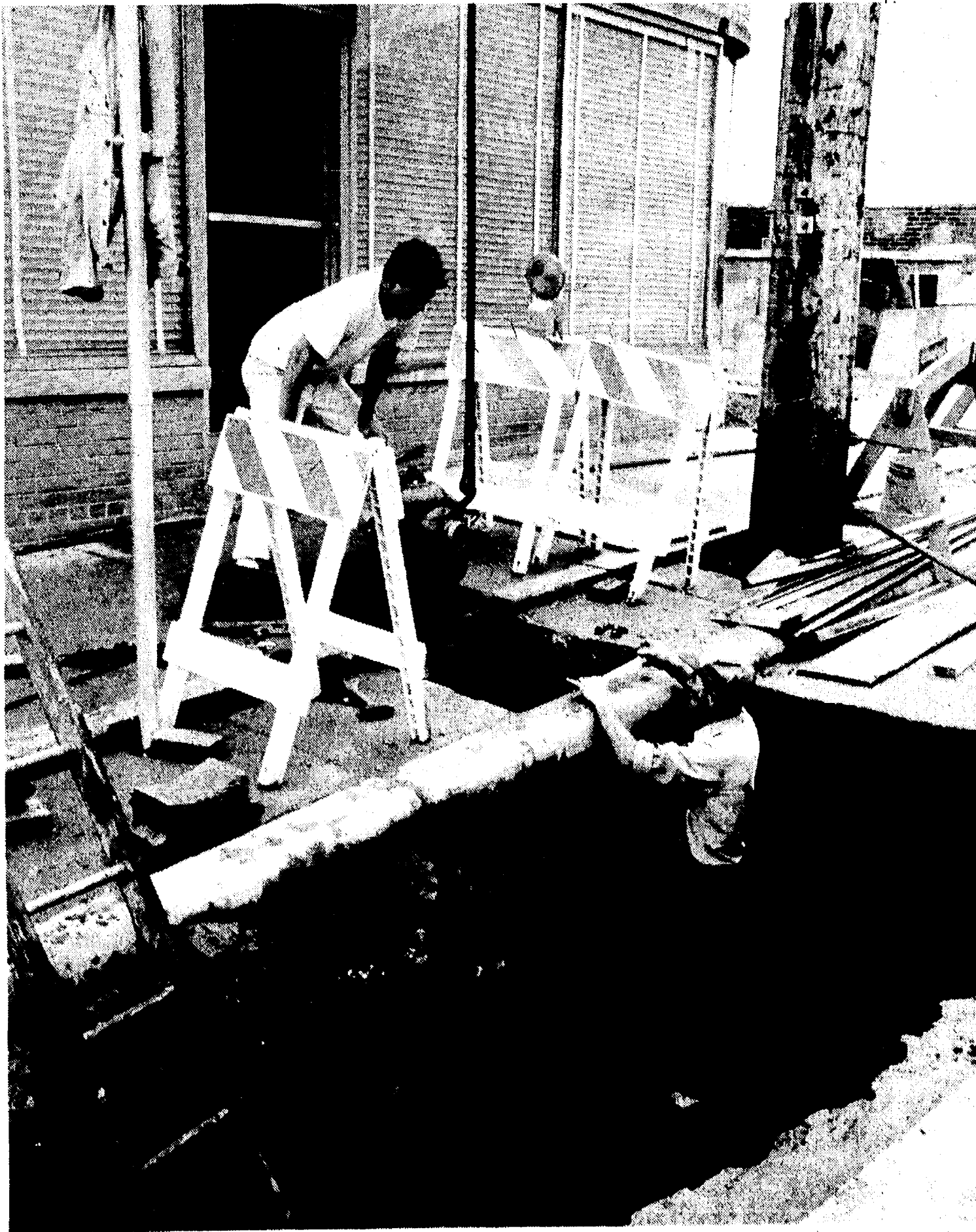
A SMALL PART OF THE WATER SUPPLY SYSTEM has been re-routed in order to serve the Sylvan Hotel building, which is being renovated for office and retail
